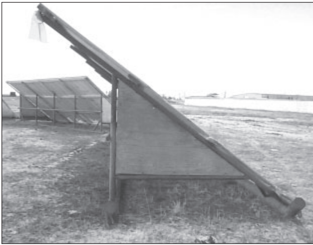
Figure 9. This slanted wall design has a railing on the back so young animals can be bedded underneath. The cross braces are welded 18 inches high so they do not become embedded in the manure pack.
