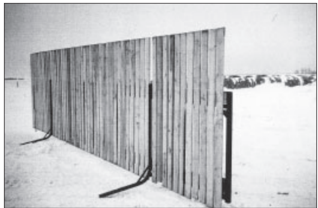
Figure 4 (top & bottom). This design requires the least amount of steel tubing in the frame. The horizontal wooden planks are not fastened to the frame, but are held in place when the slabs are nailed to the planks. The base is elevated with only four points touching the ground, reducing the possibility of freezing-in.
