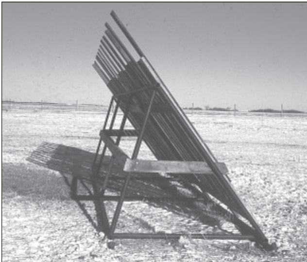
Figure 10. This slanted wall design unit overturned in 90 km/h wind gusts from the back side. For added safety, it requires extra weight or a wider base.
